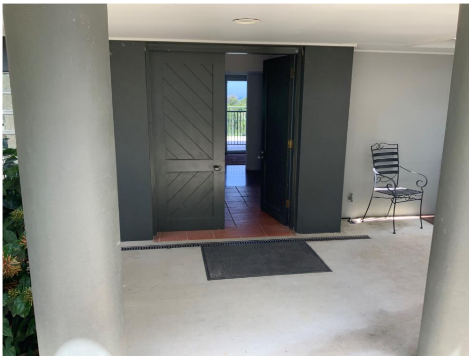
Clear access to the front double doors, with opening width of 1610mm.
